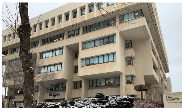
Figure 1. Image of the Provincial Law Court of Alberta. Its blocky exterior and limited visibility make it appear fortress-like. Image taken on November 28, 2019.
